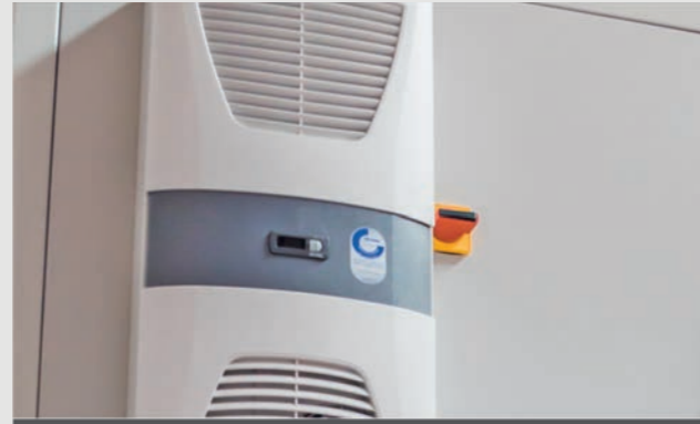
Electrical Cabinet Cooler
